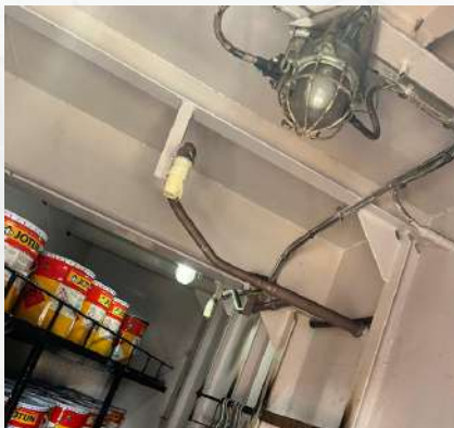
Paint room water sprinkler closed with tape.
